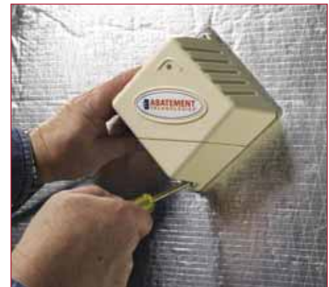
The CAP500 can be installed on duct board using the duct board adaptor plate.
